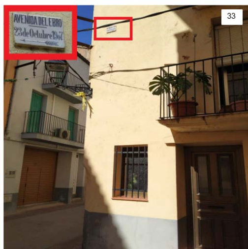
Figura 34. Carrer Federico Garcia Lorca, 14, 43512 Benifallet, Tarragona (Font: Costa J., 2021)
